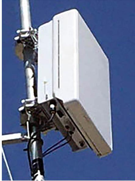
Figure 21. A MIMO 64T64R transmitter-receiver box for 5G base station. It is an integrated, weather-sealed unit with connectors on the lower edge for power and data.
